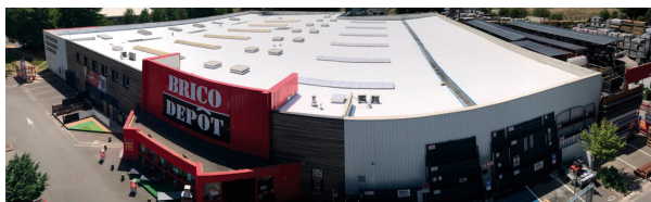
Cool roof Saumur
